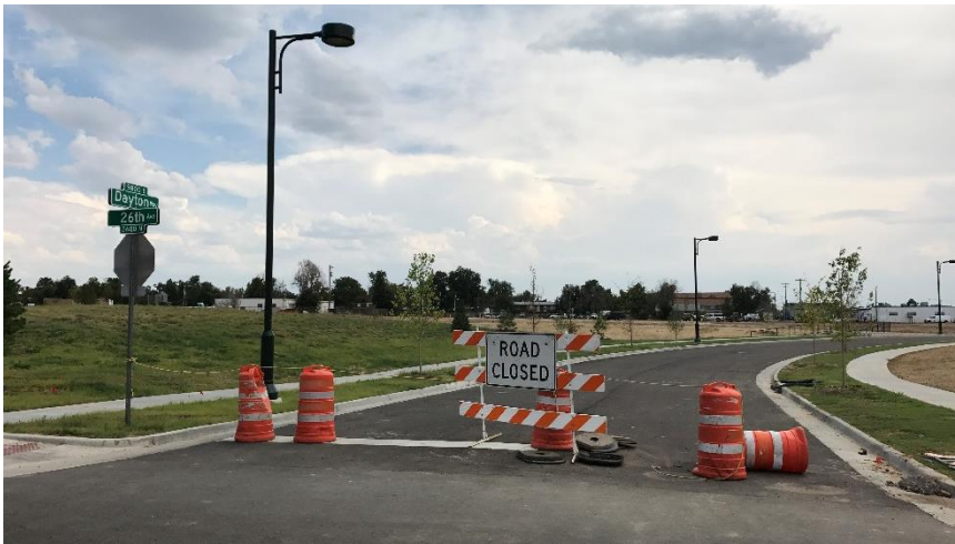
Recently constructed intersection of Dayton Way and 26th Avenue, connecting Northwest Aurora to Stapleton
