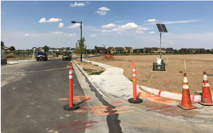
N Dayton Way connection between NW Aurora and Stapleton
